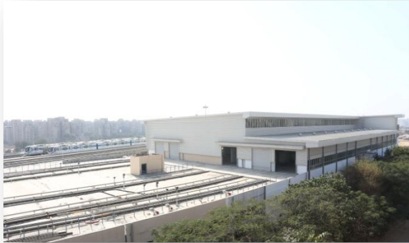
IL&FS Transportation Network Ltd (Gurgaon, Haryana)
