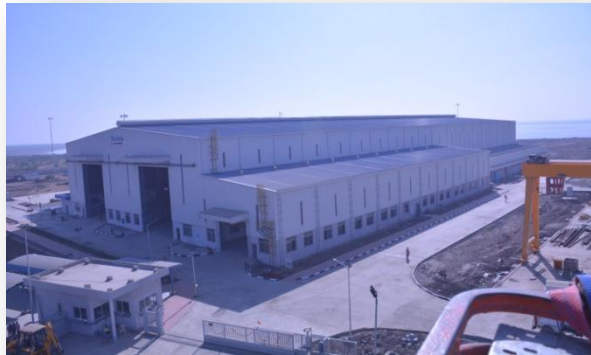
Technip (Dahej, Gujarat)
